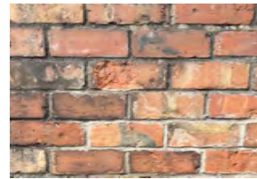
Red brick cladding to closely match existing
