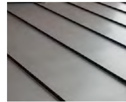
Standing seam metal roofing / cladding
